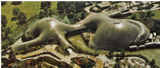
Mannheim Multihalle Gridshell
